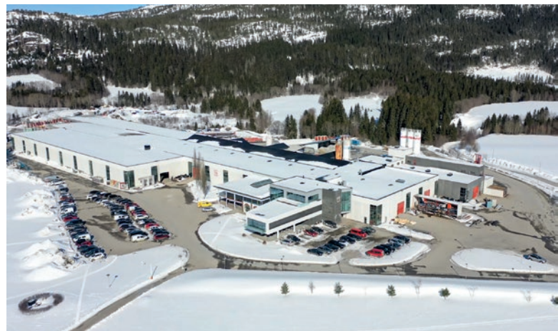
The precast plant in the town Overhalla is producing building materials since the 1940's.
